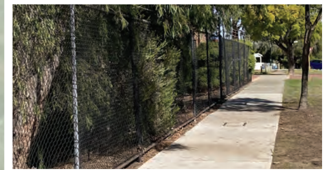
1800mm CHAIN LINK FENCE TO MATCH EXISTING
