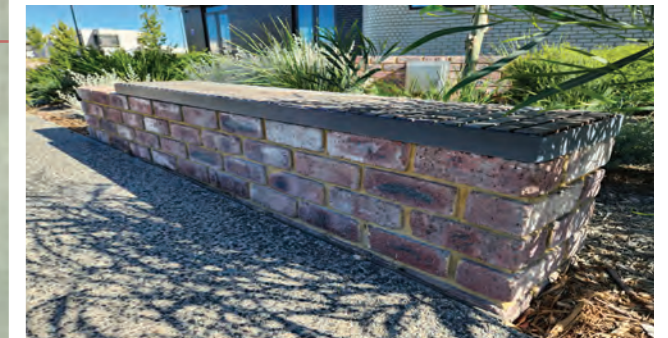
FREE STANDING WALLS TO EDGE OF GARDEN BEDS CREATE SEATING OPPORTUNITIES CAN BE USED TO RESTRICT VEHICLE ACCESS. OPPORTUNITY TO RECYCLE BRICKS FROM EXISTING BUILDING
